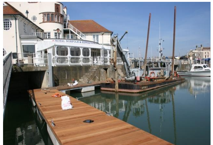
Fitting the new pontoons
